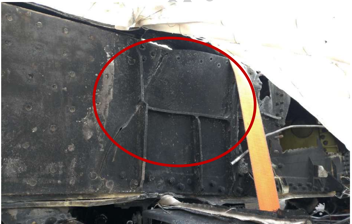
Fig. 14. The destruction of the rear spar of the left wing adjacent to ribs 5-6 and the landing gear beam hinge bracket
